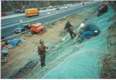
sion the system onto the slope. Lime, fertilizers and seed are placed prior to the erosion control mat and then finally the tecco mesh is installed and tensioned to the soil and rock anchors that have been drilled and grouted.
