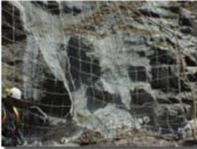
Wire mesh is used when the slope is highly weathered and/or a new slope that will weather quickly, and small rock will continuously unravel from the slope. The most effective technique for wire mesh is to drape the mesh on the slope and allow the material to make its way to the base of the slope.
